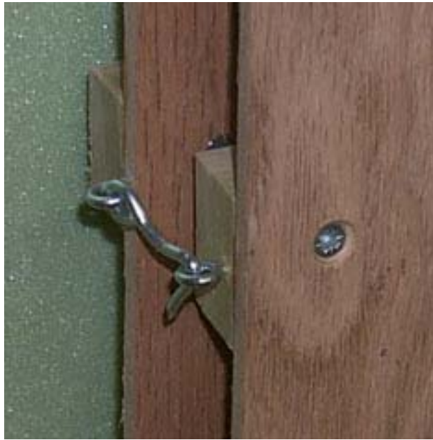
A simple hook latch secures the legs so they won't come flying out when transported.
