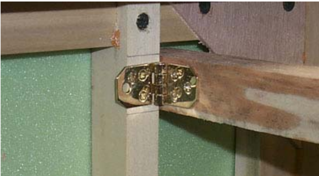
A close up view of the hinge used to attach leg pairs.
