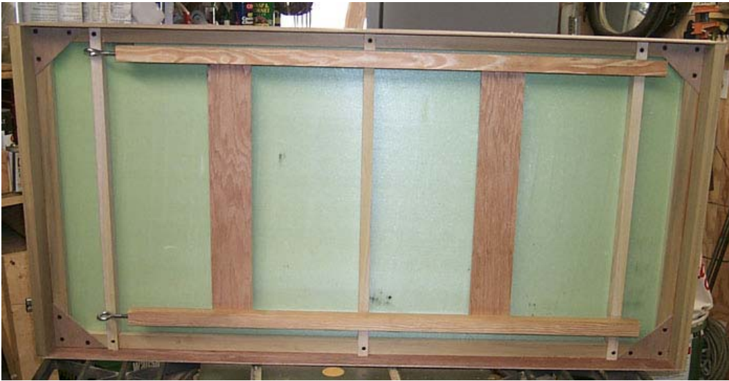
The first pair of legs is attached using hinges. Note that the braces are on the back side of the 5/4" legs.
